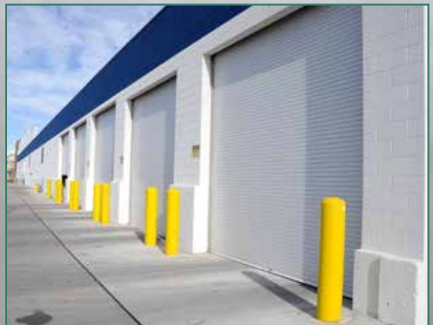
Warehouse Rolling Shutters
